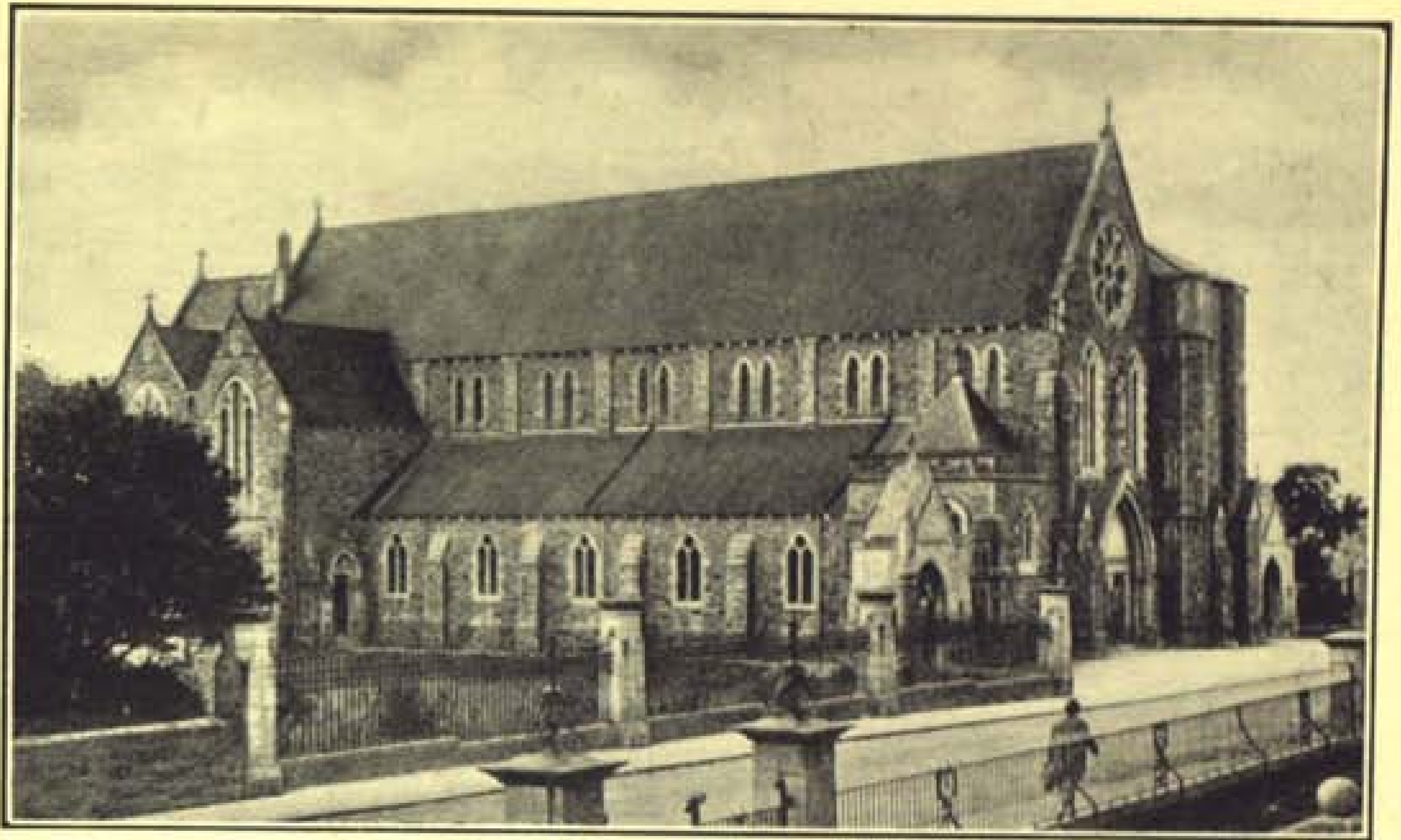
CHURCH OF THE ROSARY, CASTLEBAR.
