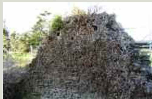
*The top layer of vegetation has been sprayed and killed off pending its removal. The treatment allows for assessment and recording of the masonry*
