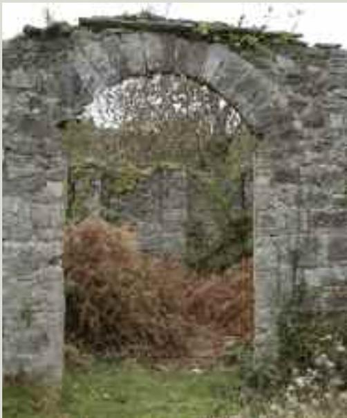
*Arch over a door opening. This arch is also vulnerable because the wall over the arch has been lost*
