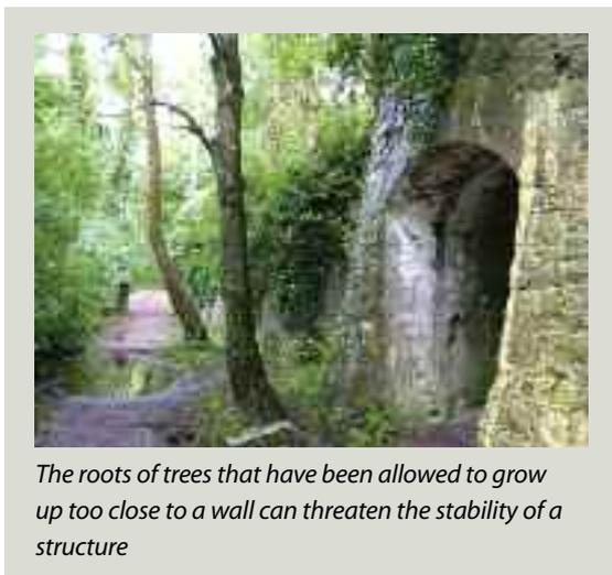
*The roots of trees that have been allowed to grow up too close to a wall can threaten the stability of a structure*
