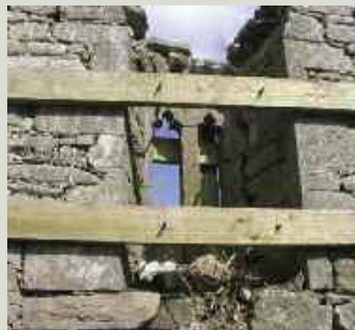
*Timber bracing in the vertical plane to secure a window opening where a collapse outwards was imminent. The temporary work consisted of planks bolted through the opening*
