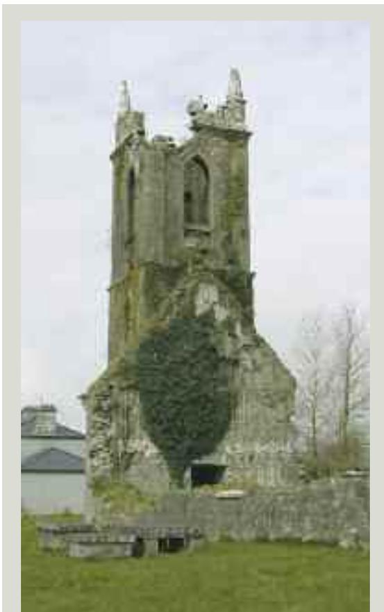
*Ruins are often found in isolated areas and a structure such as a tower may be the tallest in its locality making it vulnerable to lightning strike. The tower of this ruined church was struck by lightning which destroyed the corner pinnacles*
