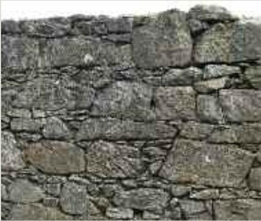
*The small stones used as pinnings can be easily lost as the mortar holding them in place erodes over time. When repairing a wall, it is important to collect any fallen pinnings and reincorporate them into the joints as they are an essential characteristic of the wall*
