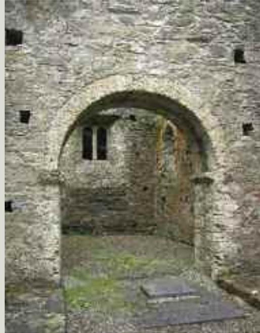
*Putlog holes, literally holes in a masonry wall where timbers were put, are a common feature of mediaeval buildings*
