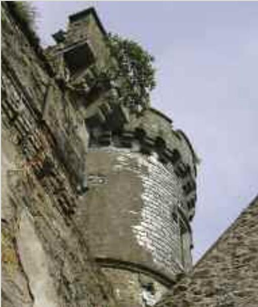
*While more commonly found as a roofing material, slate was also used as a cladding material for exposed walls, gables and chimney stacks. The slates found in slate-hanging are often rare examples of native Irish slates which, because of their small sizes, were often replaced on roofs by Welsh slates*
