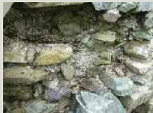
*Wall with its outer face lost exposing the construction of the wall core*
