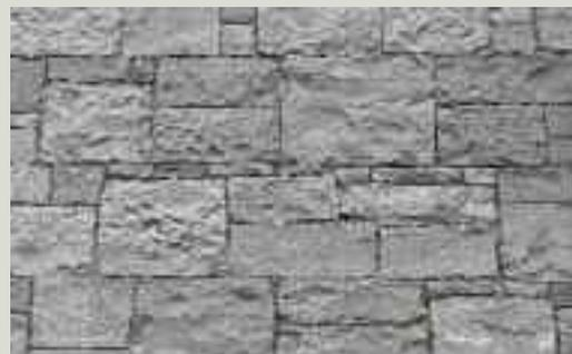
*Sneaked masonry, sometimes called random ashlar, was built in discontinuous courses with small stones or snecks introduced to break courses. The stones required cutting but offered economy in material as smaller stones could be used. This style of construction was first used in the nineteenth century and is distinctly Victorian*
