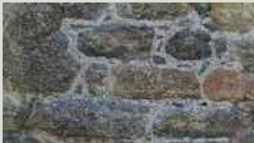
*A mediaeval wall repointed with pinnings used in the larger joints*
