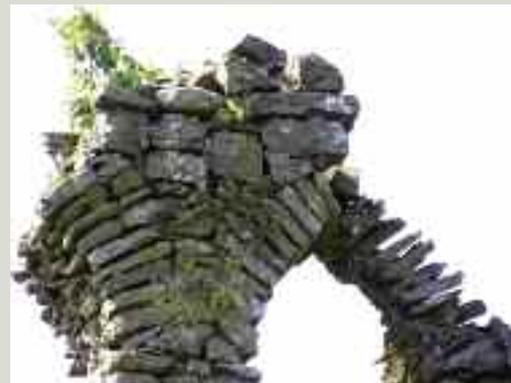
*One arch on this double bell-cote has already failed. The other is on the point of collapse due to loss of mortar through erosion and exposure*
