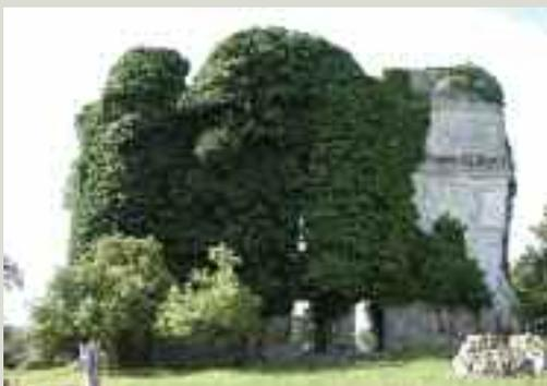
*Vegetation which is allowed to grow unchecked can rapidly overwhelm a structure and accelerate its decay*
