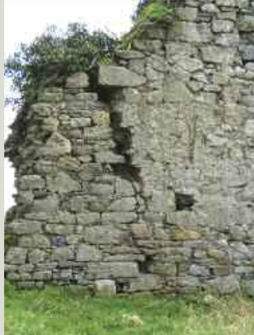
*Tapering cracks can result from subsidence. As the crack widens the smaller stones fall out or drop inside the wall creating a wedge effect and increasing the damage*
