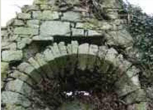
*Arch over a window. Note the damage done by the improper removal of ivy which pulled out the smaller packing stones and has left the arch vulnerable*
