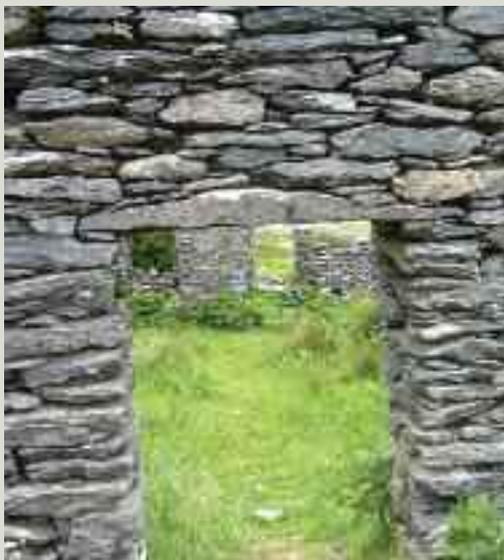
*Stone lintel over a narrow opening. The thinness of the lintel, particularly at the right-hand end, makes it vulnerable to cracking*
