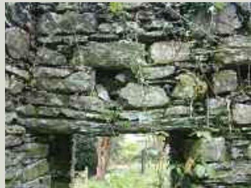
*Lintel failure in this case was probably the result of the loss of mortar and stone from the wall above the lintel which damaged the natural self-arching tendency of the masonry placing excessive loading onto the lintel*
