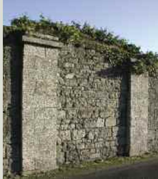
*This image highlights the contrast between the finely worked stonework of the ashlar piers, with narrow joints between the stones, and the coursed rubble walling that was used to block up the former gateway between the piers*
