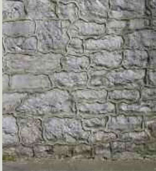
*Strap pointing is a style of pointing which must be avoided on historic masonry structures. Unfortunately, it is quite a common intervention and was often used where the original joints were very fine. Unsightly and damaging to the stone, the pointing is proud of the stone surface and traps water on the ledges formed. It also partially adheres to the face of the stone and is almost always cement-based*
