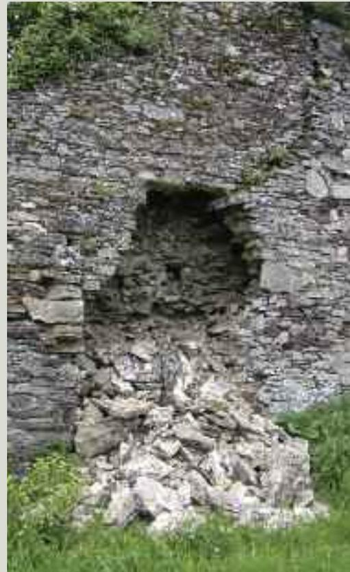
*A partial collapse of the town wall of Youghal, County Cork. Recently-collapsed structures should not be approached until after a structural engineer has deemed it safe to do so*
