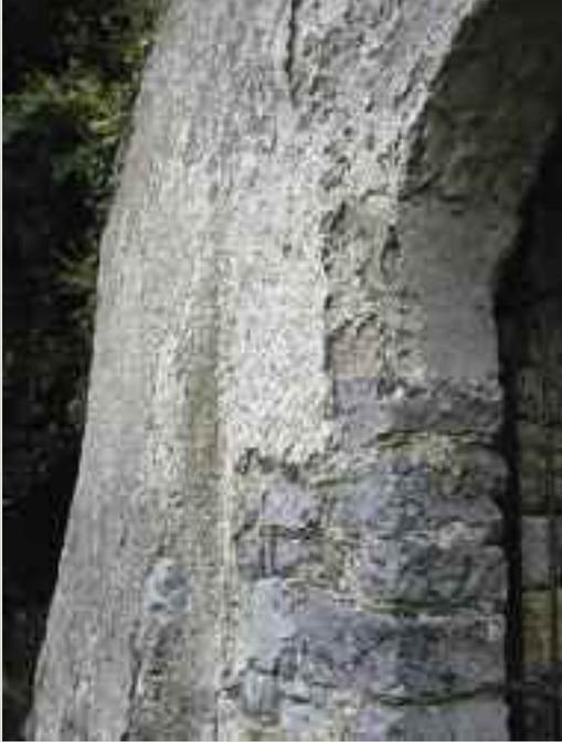
*A wall showing surviving traces of external lime render. Most rubble-walled buildings were originally rendered to keep rainwater from penetrating into the interior*
