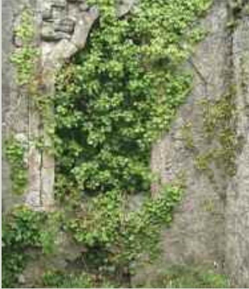
*Ivy can become established within a masonry wall, growing unchecked through the joints and re-emerging in other parts of the structure*
