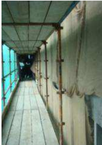
Cosaint heiseáin ar oibreacha aoil
