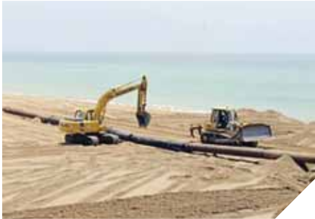
Forte Novo - reloading the Garrão foreshore, 2010 (Portugal)
