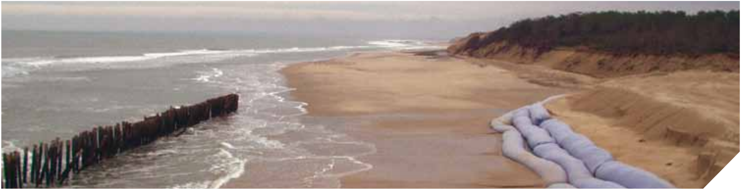
Hydraulic piling, Cap Ferret, Aquitaine (France)
