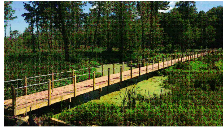
BOARDWALK OVER WETLAND
